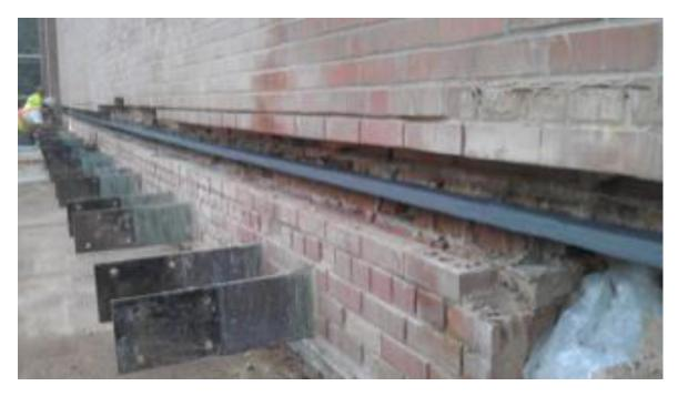
Current examples of brick flaking and brick efflorescence on the sanctuary walls.
